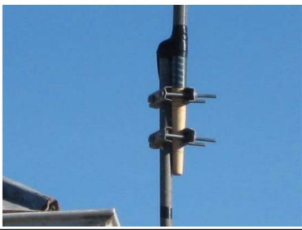
With the u/v bolts, washers and nuts the pipe and rod were joined together. Thanks to Jim Searle.
